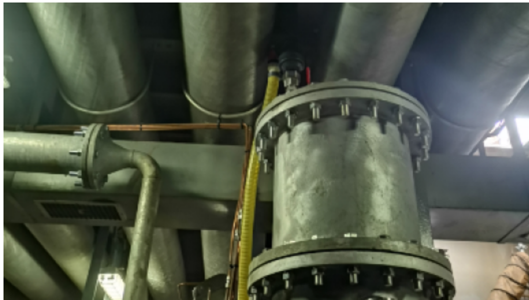
2 x 1000 cubic meters ballast water treatment system inside of a semi-sub barge.
